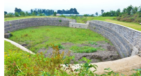
Picture: One of the Check dams constructed at the base of Mount Muhabura. Source : Tubibe Amahoro.
